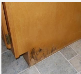
OLD DAMAGE W/MOLD
